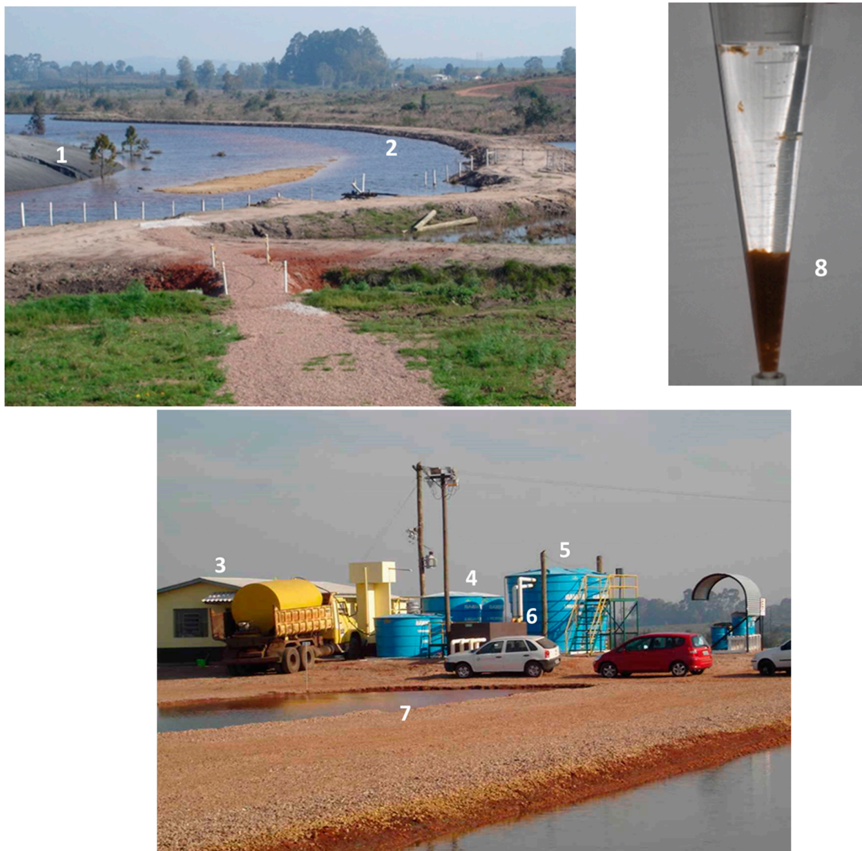
Figure 3. Photographs of the Capão da Roça coal waste site taken in 2010, Charqueadas county, Rio Grande do Sul, Brazil: (1) coal waste deposit, (2) dam for acidic water retention, (3) laboratory, (4) preparation of reagents in containers, (5) mixing tanks, (6) baffled flow unit for the formation of flocs, (7) settling ponds, and (8) results of the chemical neutralisation process shown in an Imhoff cone.
